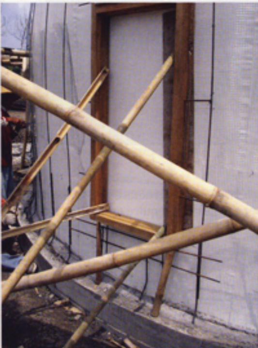
Fig. 3: A wood-framed window opening braced in place before placing concrete. Additional reinforcement will be placed around this and other openings in the dome
