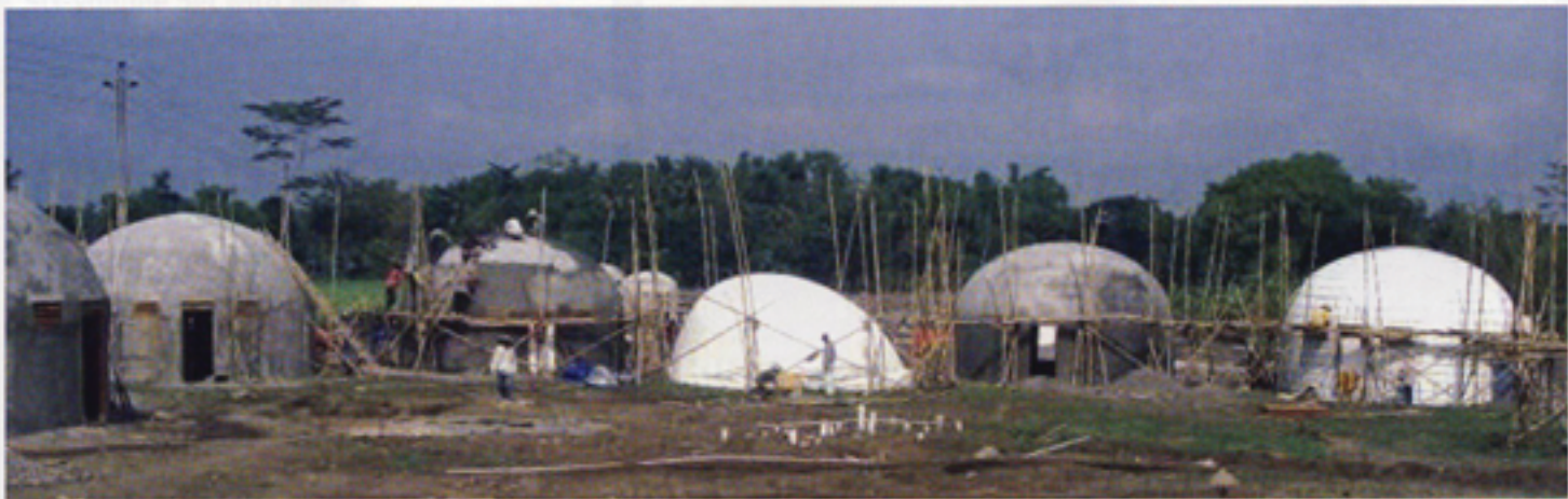
Fig. 4: Panoramic view of New Ngelepen construction shows several homes in various stages (from the left): A dome with the shotcrete hardened, a dome with most of the concrete applied and the crew still working at the top, an air form being inflated, a dome with the concrete completed and in the process of curing, and a fully inflated form with much of the reinforcement in place
