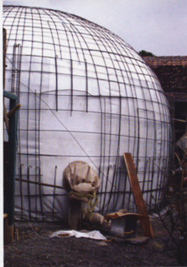
Fig. 1: Inflated form with most of the reinforcement installed. The small fan used for inflation remains in place, connected to the fabric of the form
